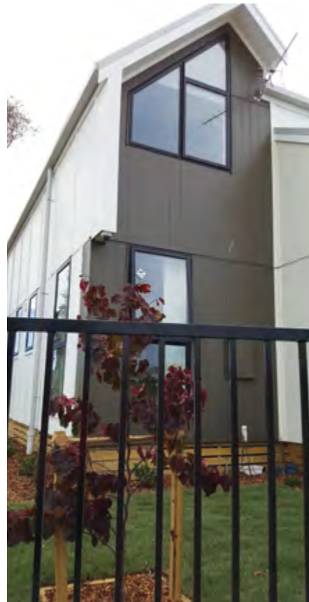
A much-welcomed new Housing New Zealand development in Aranui will be tenanted by families this month.
