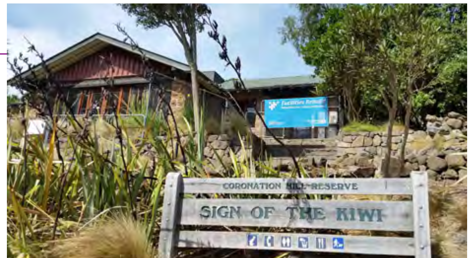
Repair and restoration of the historic Sign of the Kiwi are underway.
