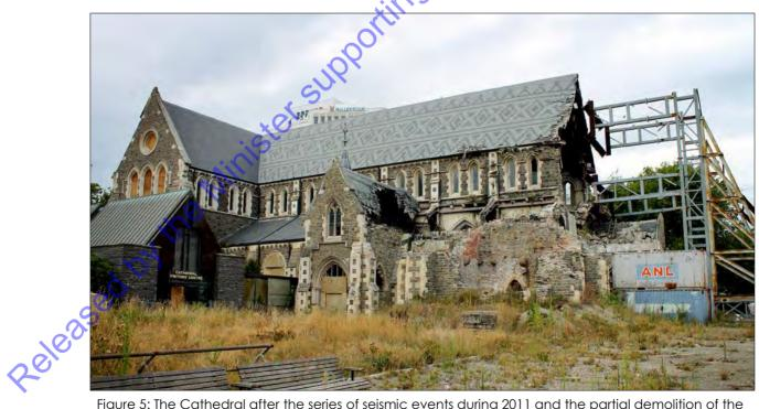
Figure 5: The Cathedral after the series of seismic events during 2011 and the partial demolition of the tower. *Photograph: http://www.vengavalevamos.com/2016/03/christchurch-new-zealand/*
