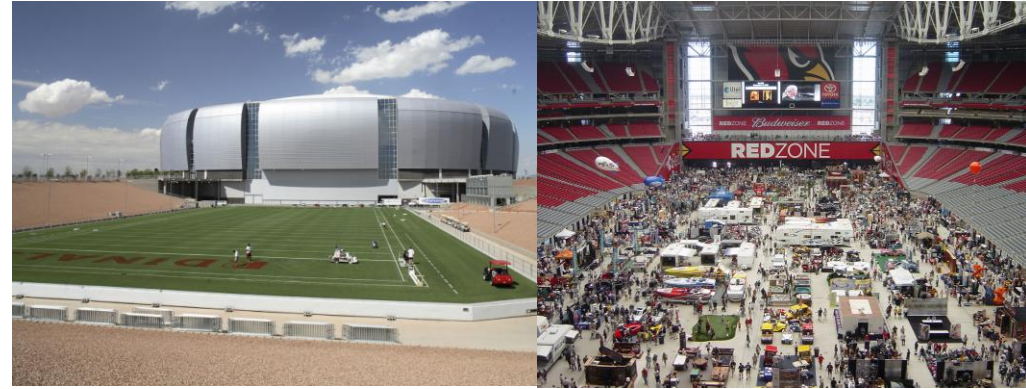
University of Phoenix Stadium
