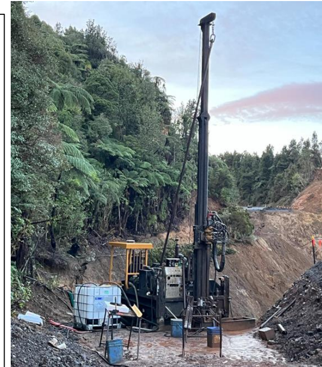
Construction begins on the bridge reconnecting SH25A in the Coromandel
