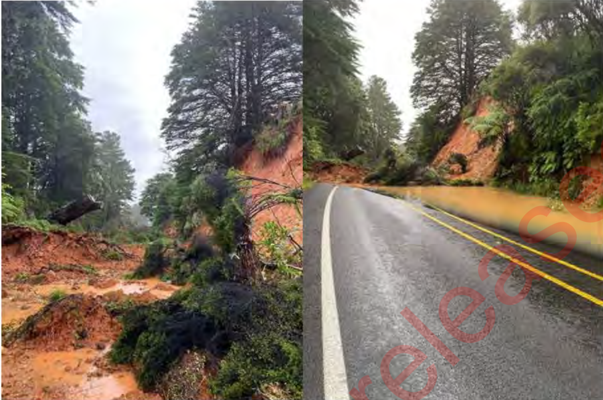
State Highway 1 at Puhoi
