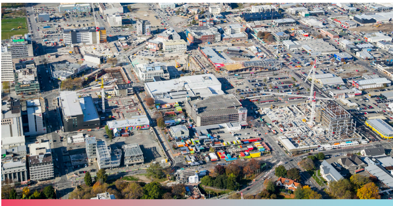
Aerial view of public and private developments, May 2015
