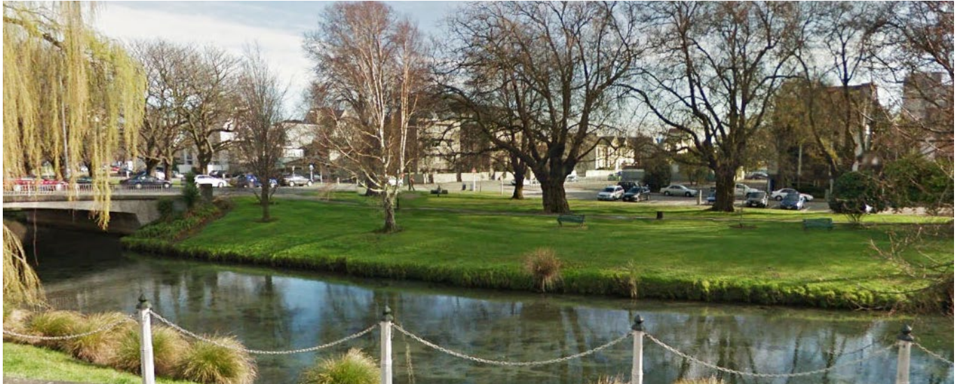
3 From Oxford Terrace, looking north, Montreal Street bridge on the left.
