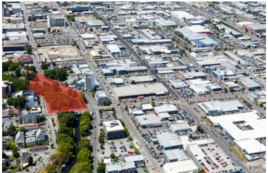
▲ Aerial view looking east
