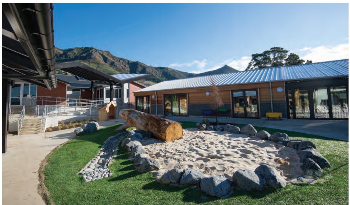
Cholmondeley rebuild celebrated. Image courtesy of RMBH Architects. Photography by Centuri Chan.
