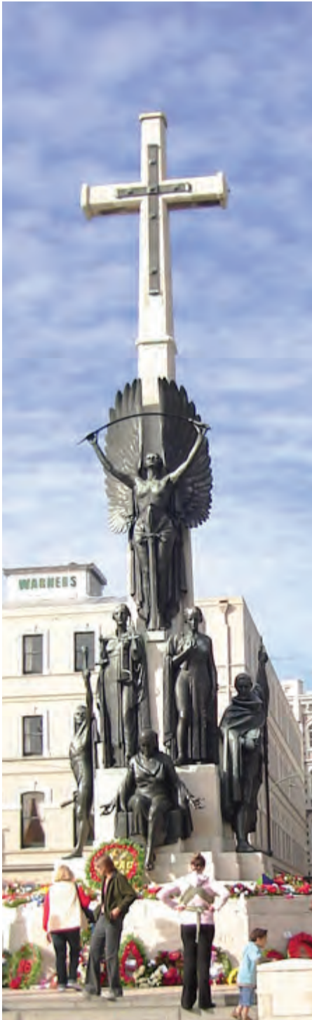
Investigation work needs to be done on the Citizens' War Memorial in Cathedral Square to determine the best repair strategy.
