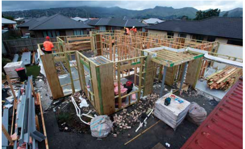
Houses being broken down and flatpacked. The innovative new technique recycles and re-uses newer houses that would otherwise be demolished.
