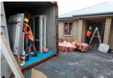
Houses being broken down and flatpacked. The innovative new technique recycles and re-uses newer houses that would otherwise be demolished.
