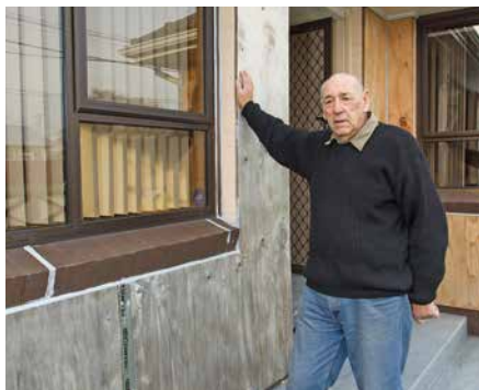
Len Smith examines the temporary repairs to his badly cracked windows.
