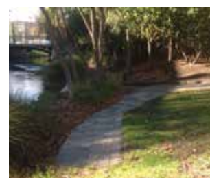
29 Earthquake slumping damage and unusable ground condition.
