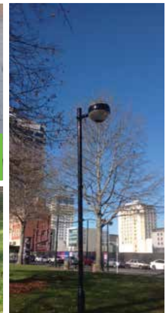
Unable to get new parts to repair and maintain existing light fittings.
